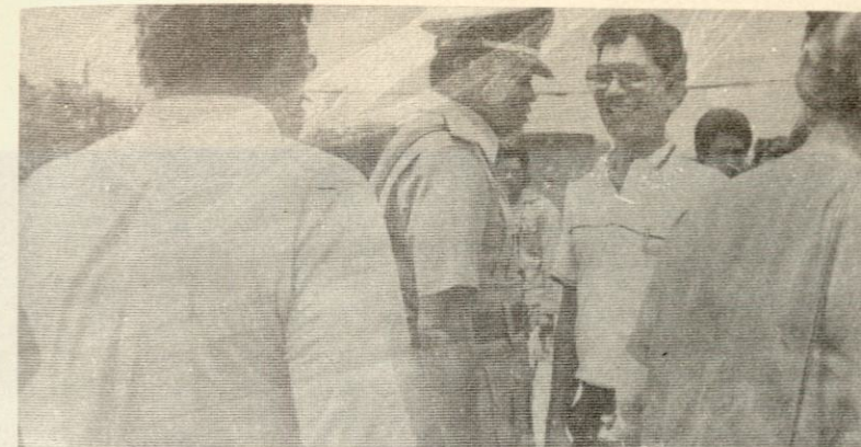
Brig. Gen. Prospero Olivas, Metrocom Chief and Director of the Integrated National Police, with Arch. Gerardo G. Magat, Chairman of the QC Task Force on Relocation, Resettlement and Rehabilitation. They are inspecting the on-going demolition operation at the road-right-of-way of the Don Mariano Marcos Avenue.
